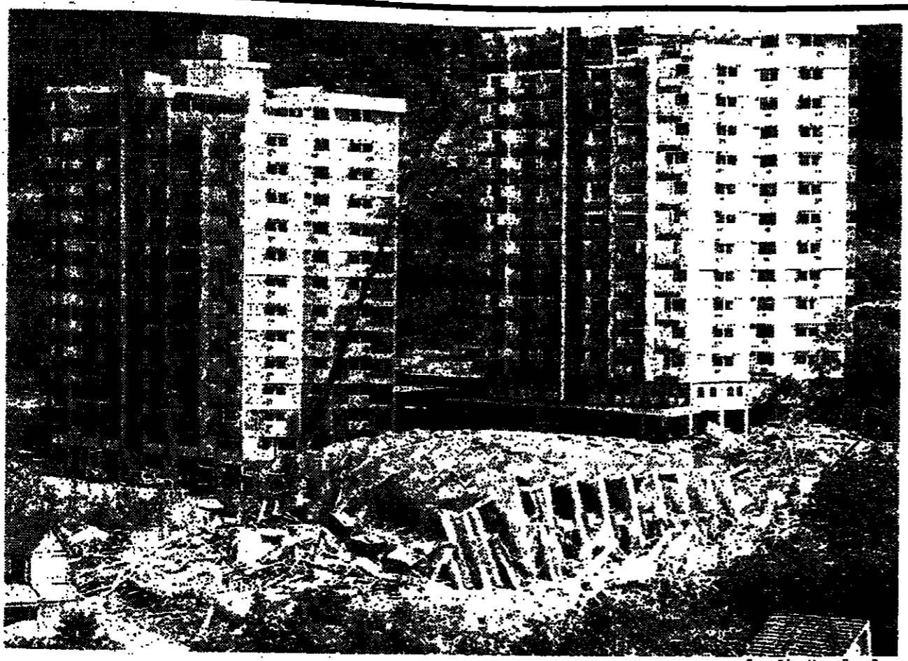
ONLY RUBBLE LEFT — A 12-story apartment block outside Kuala Lumpur collapsed after it was hit by a landslide, killing at least one person. About 50 people were believed trapped in the ruins. Nearby apartment blocks have been evacuated as a precaution. A consortium signed a contract last month to build twin 85-story office towers in the city that would be among world's tallest.
